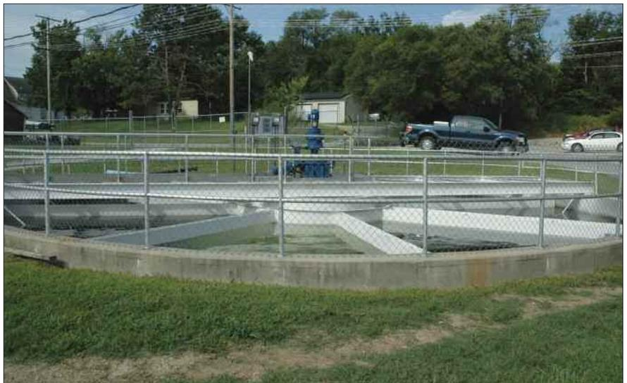
A new center shaft, drive mechanism, and troughs were installed in the existing clarifier. The center shaft of the original clarifier failed while rehab work was being done on other parts of the plant.
