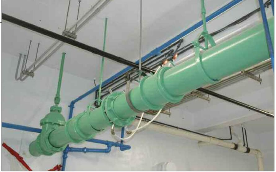
This photo shows the line with the static mixer with a section of line with mixing elements installed inside the pipe. The static mixer is a replacement for the flash mix unit which has been bypassed and will not be used.
