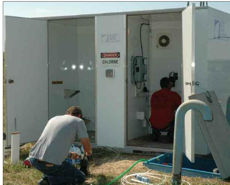
**KRWA has installed rechlorination stations in various water systems to help them maintain chlorine residuals. This photo shows KRWA's Tony Kimmi and Lonnie Boller working to make connections to a RWD's pumping station.**
