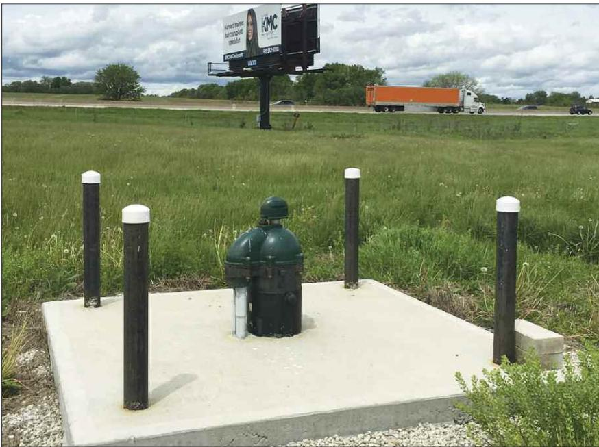
**Suburban Well No. 13 was drilled in February of 2018 by Sargent Drilling, to replace a battery of shallower wells. This well and its water rights were purchased by Leavenworth RWD 7 in 2019.**
