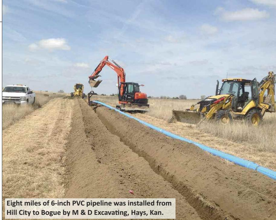
Eight miles of 6-inch PVC pipeline was installed from Hill City to Bogue by M & D Excavating, Hays, Kan.
