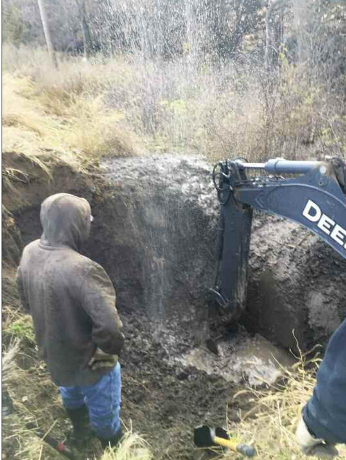
**Repairs starting on the 80 gpm leak that was located at the end of a farm field.**
