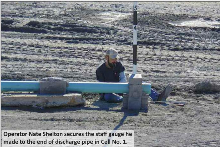
**Operator Nate Shelton secures the staff gauge he made to the end of discharge pipe in Cell No. 1.**
