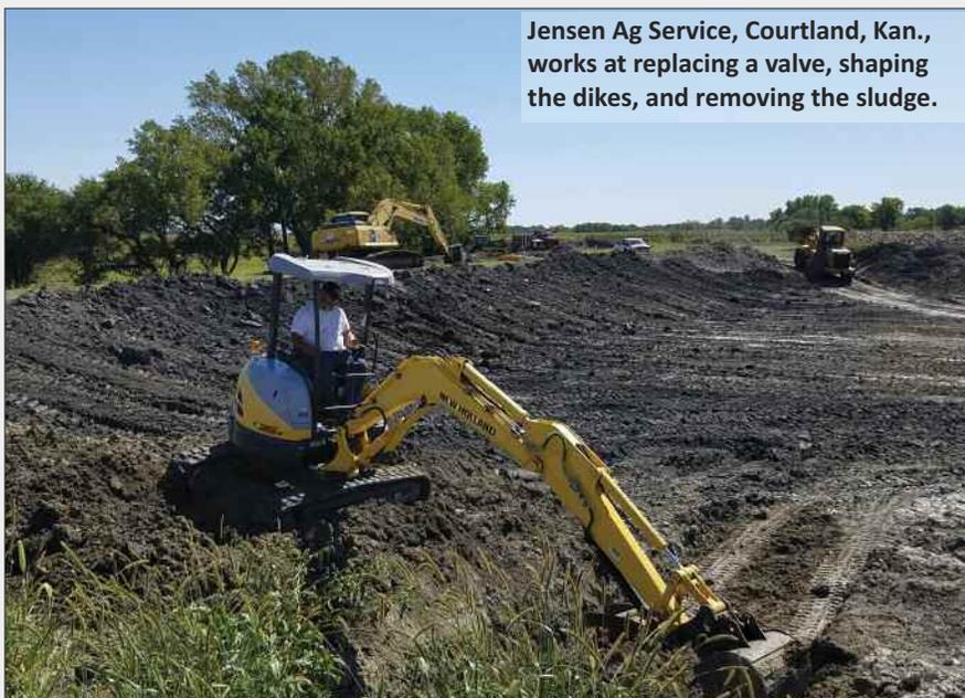
Jensen Ag Service, Courtland, Kan., works at replacing a valve, shaping the dikes, and removing the sludge.
