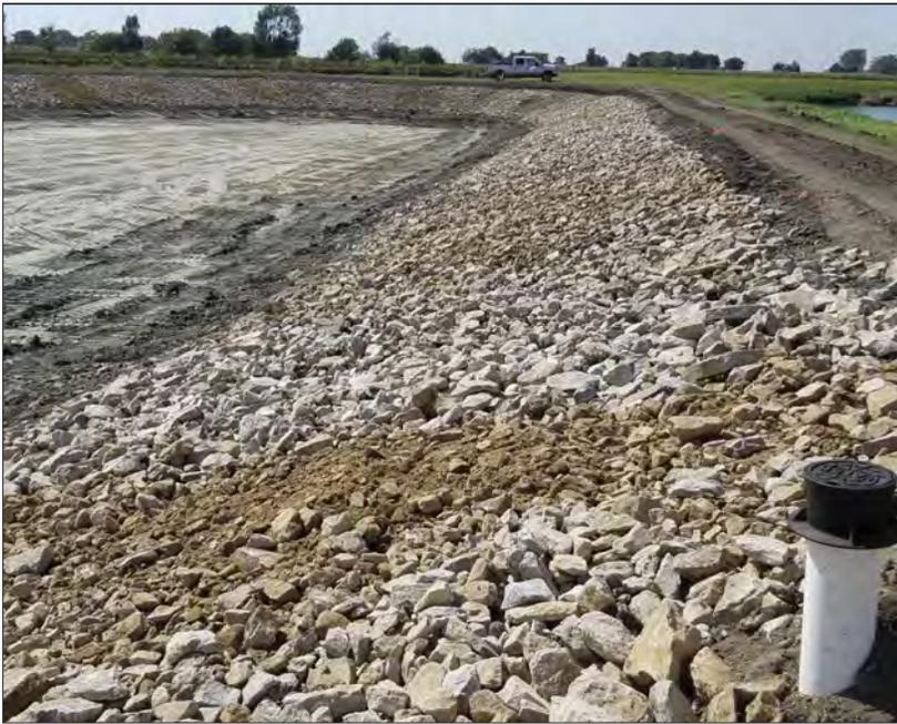
This photo shows the a second of lagoon dike that was repaired and after rip rap was added.
