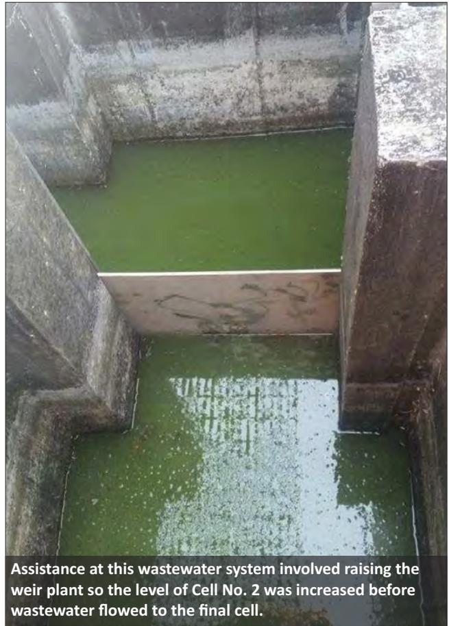
Assistance at this wastewater system involved raising the weir plant so the level of Cell No. 2 was increased before wastewater flowed to the final cell.
