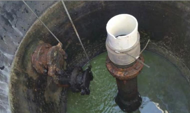
The lower discharge pipe is now being used and a short extension to ensure five feet of operating depth.
