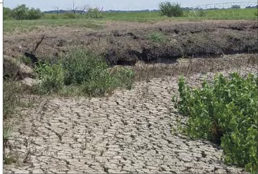
Severe dike erosion was noted when performing the sludge profile. After the cell was drained the erosion was more noticeable as shown in this photo.
