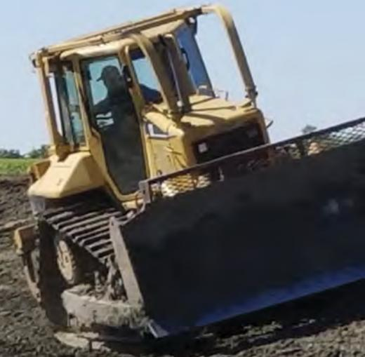
The lagoon was repaired by the city; sludge was removed and the dikes were repaired and reshaped to like new.
