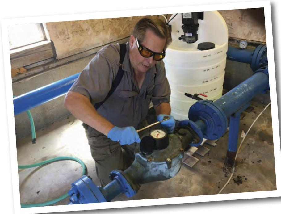
**KRWA Technical Assistant Doug Guenther works on the repair of a 2-inch meter at the city of Bison. The meter was shattered on the inside, likely due to air being pumped.**
