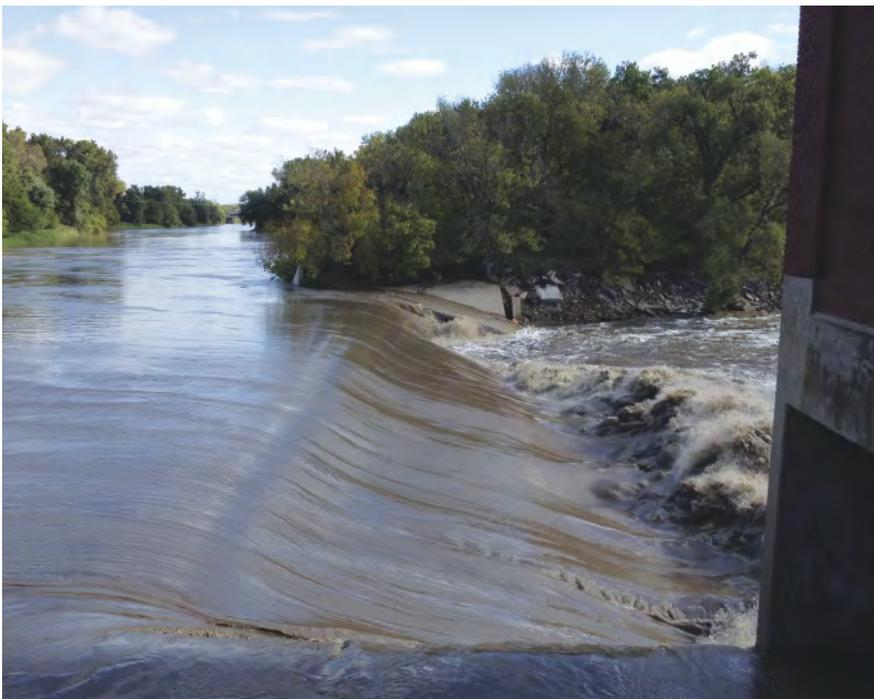
**Big Blue River as it appeared on October 3, 2014, with approximately 9,000 c.f.s. spilling over the dam. Erosion of the face of the dam is clearly evident on the far end. Streamflow over the dam on May 4, 2018, when it ultimately failed was approximately 4,000 c.f.s.**
