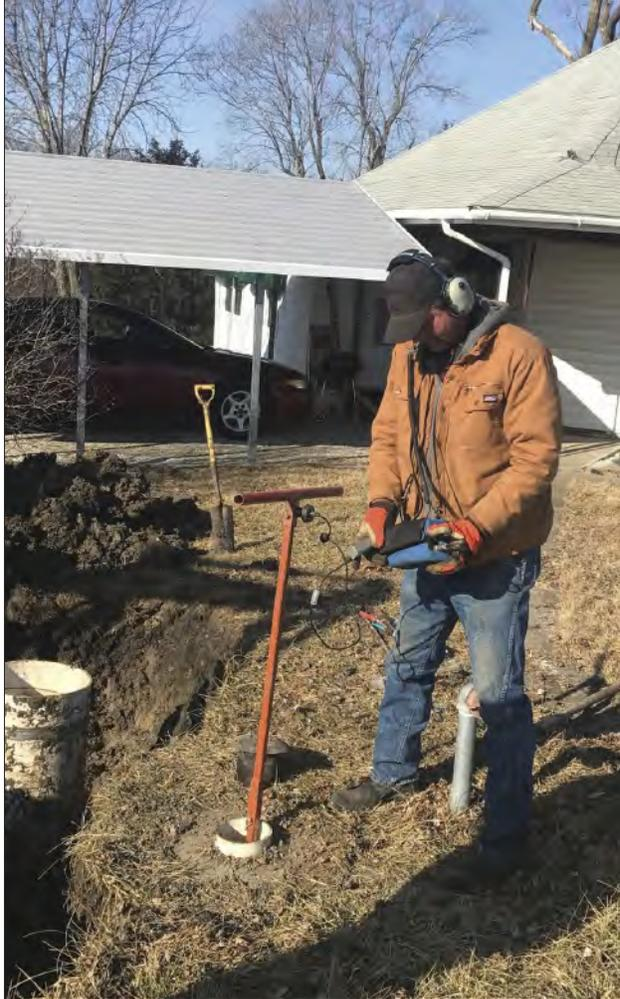
**KRWA Tech Tony Kimmi uses sonic leak detection equipment to try to further isolate possible leak on service line to this customer.**
