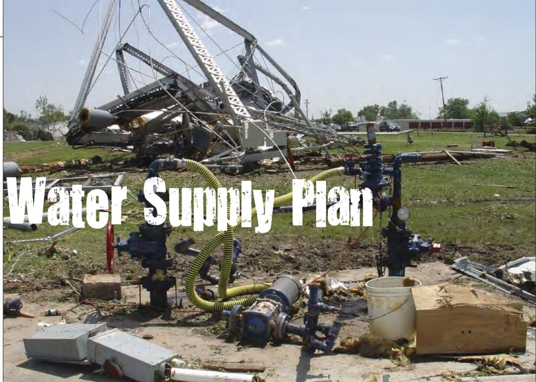
The city of Jewell's elevated storage tank and pump station were destroyed by a tornado May 29, 2008.
