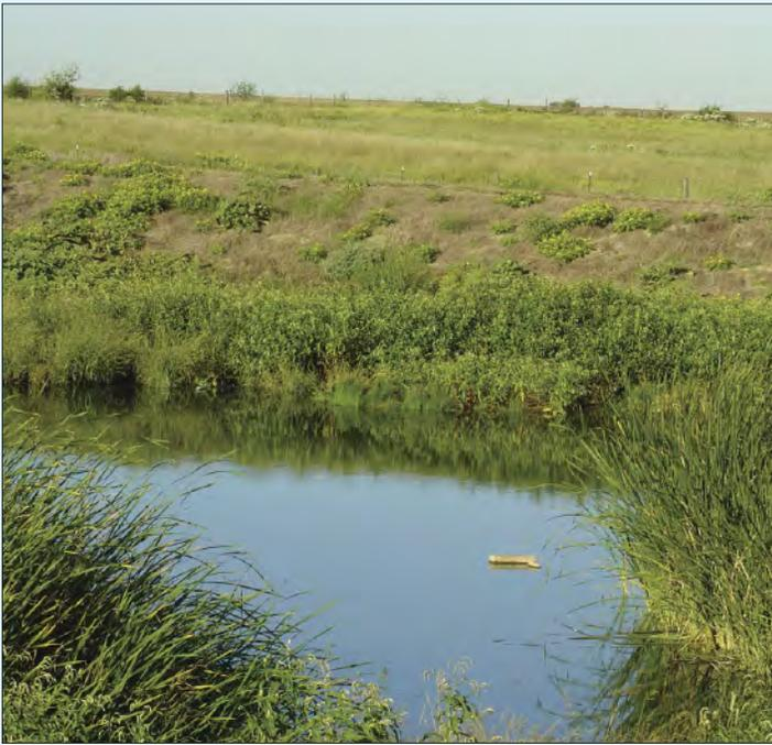
**Cattails should never be allowed to overtake a lagoon cell as in this photo. They can cause many problems including excessive seepage due to their extensive root system. Cattails are also a preferred food source of muskrats.**
