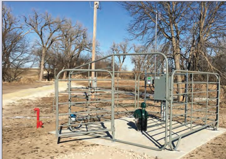
**The new municipal water supply well is located very near the irrigation well it replaced. Electrical service was already present, and the properties of the aquifer at that location were known to be satisfactory. The well is not located in a cultivated field and the irrigation well that was replaced has been plugged.**
