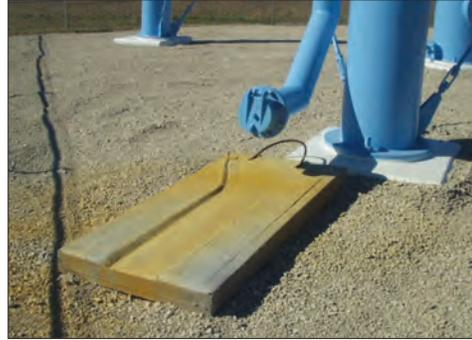
**This is the overflow line on an elevated storage tank. Note the flapper-gate at the end of the overflow to prevent the entrance of vectors. A splash pad has also been provided to prevent erosion problems.**
