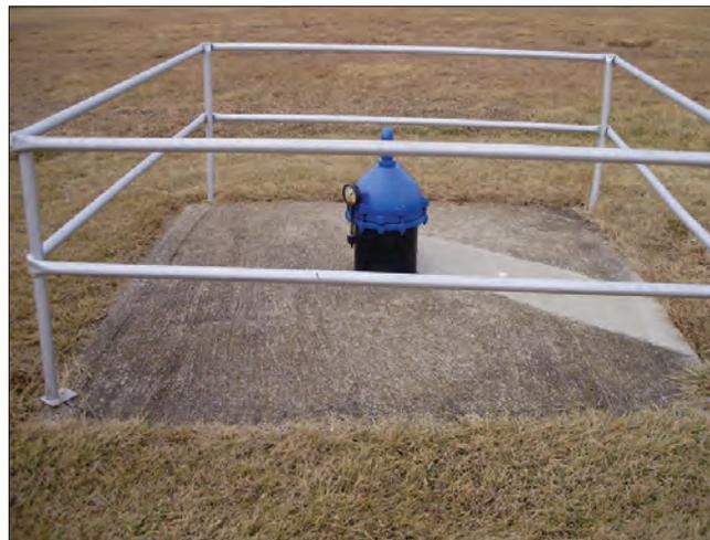
**Note this well is very well maintained with screened well vent and drawdown gauge. Also note the crack in the concrete slab that has been repaired with grout to prevent the entrance of contaminants.**
