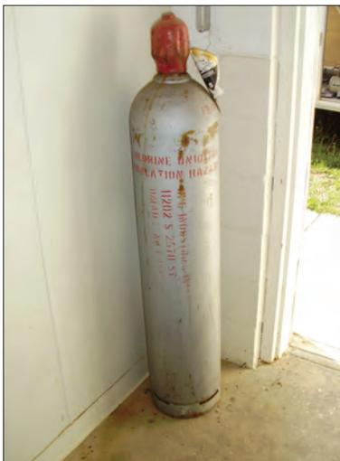
KDHE requires that all chlorine gas cylinders be restrained with a chain, whether empty or full. Note this cylinder is not restrained.
