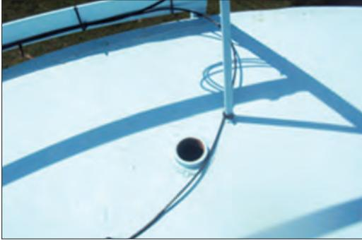
**Notice the opening on top of standpipe. This opening allowed birds to enter the standpipe, but they could not escape. They eventually died, contaminating the water within the standpipe.**
