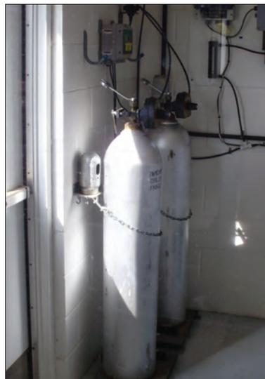
The photo shows a chlorine gas cylinder with proper chain restraint and wrenches on shut-off valves.
