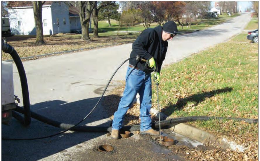
City of Effingham, Kan. operator James Ellis operates the power washer to clean an additional waterline valve riser.
