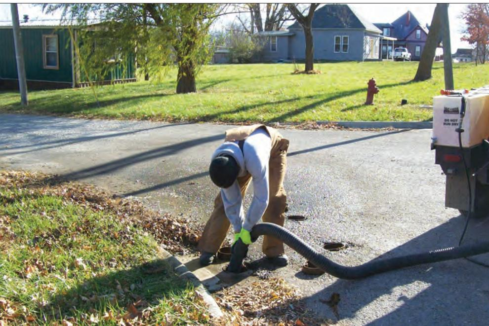
Valve riser being vacuumed prior to exercising the valve.
