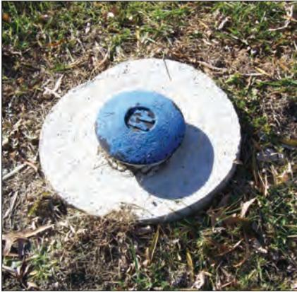
This freshly painted valve riser cap indicates the valve was exercised and is operable.
