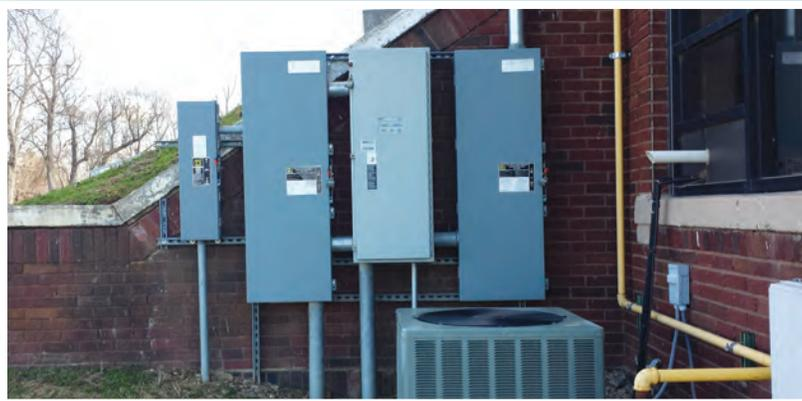
Eric Boone, City Superintendent at Yates Center, Kan. checks the standby generator at the city's water plant. The controls show the disconnect and transfer switch arrangement.
