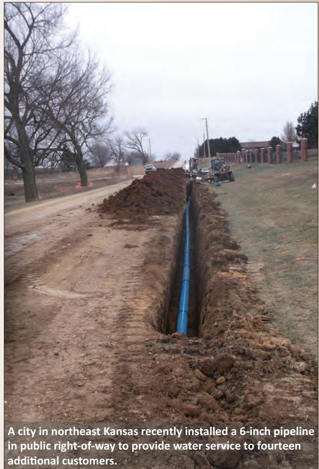
A city in northeast Kansas recently installed a 6-inch pipeline in public right-of-way to provide water service to fourteen additional customers.
