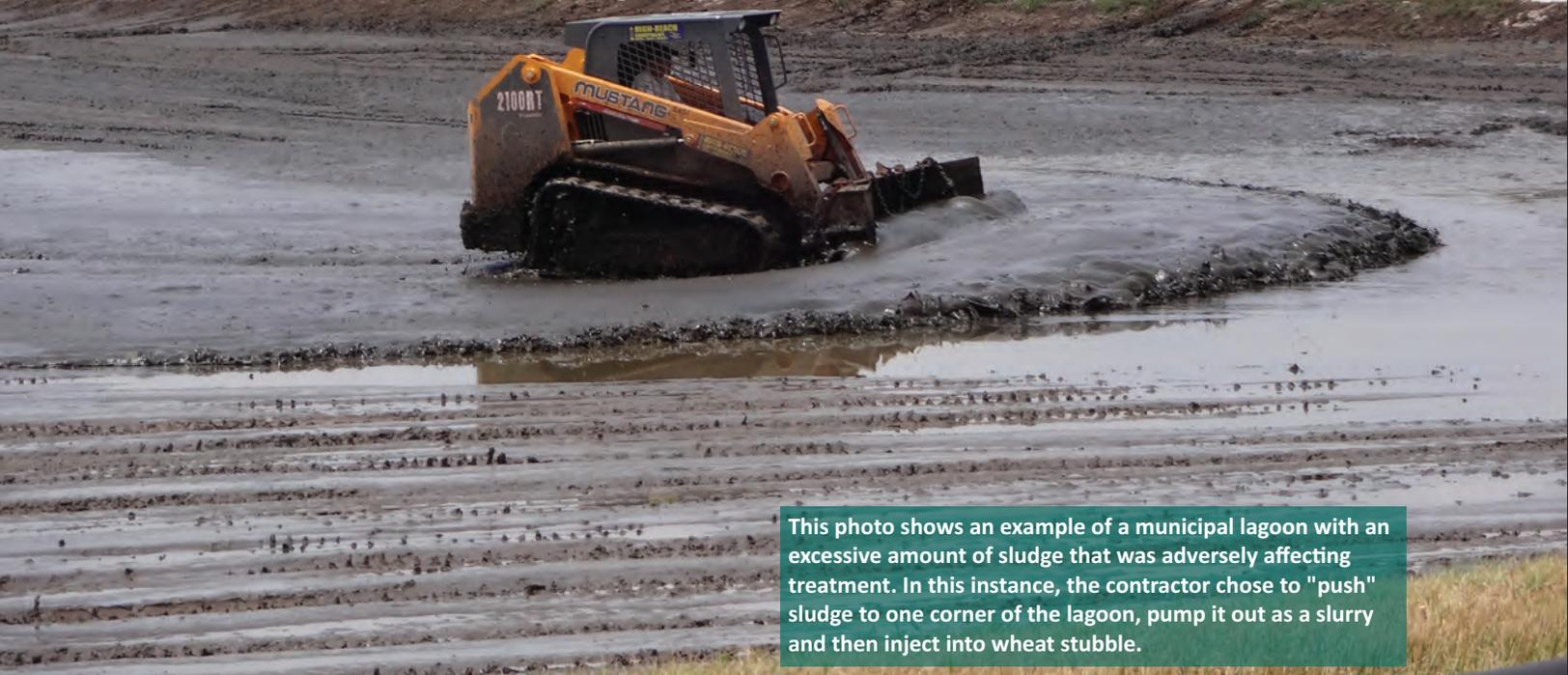
This photo shows an example of a municipal lagoon with an excessive amount of sludge that was adversely affecting treatment. In this instance, the contractor chose to "push" sludge to one corner of the lagoon, pump it out as a slurry and then inject into wheat stubble.
