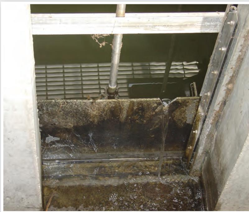
This V-notch has been cut into the top of the metal weir plate to allow for easier and more representative effluent sample collection. Note the biological growth, etc. on the plate that may have ended up in the sample prior to cutting the V-notch.
