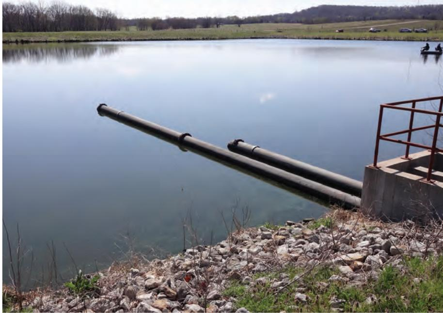
The discharge structure on the final cell of this lagoon was designed to draw effluent from two different depths in order to avoid algae near the surface. Typically the lower pipe is used during the summer and the upper one during the winter.
