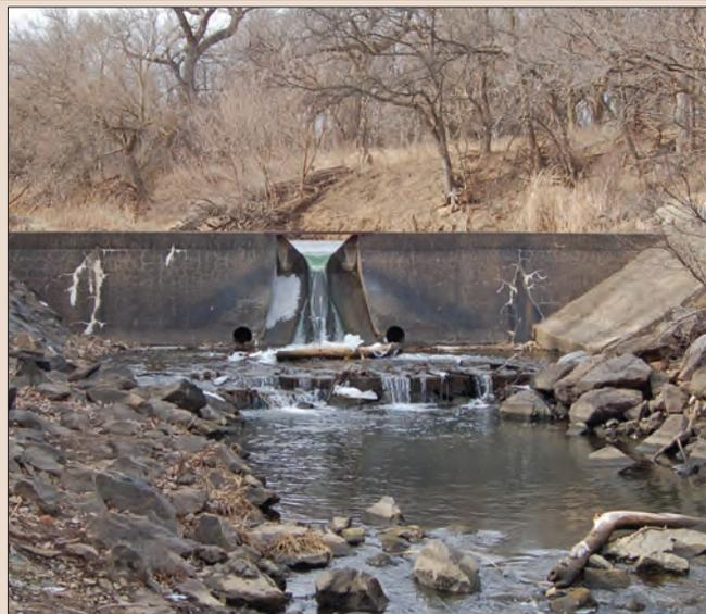
Water from the Sand Creek flows toward the Smoky Hill River and is measured at the structure commonly called the V-Notch. Discharge from the control gates takes into account the quantity water flowing through the V-Notch when adjustments to the downstream flow rates are taken.
