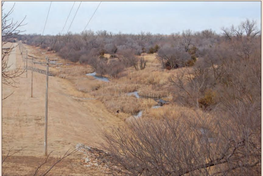
**Normal and designed-for water seepage from the Kanopolis Dam is collected and conveyed to the Smoky Hill River via a small creek.**
