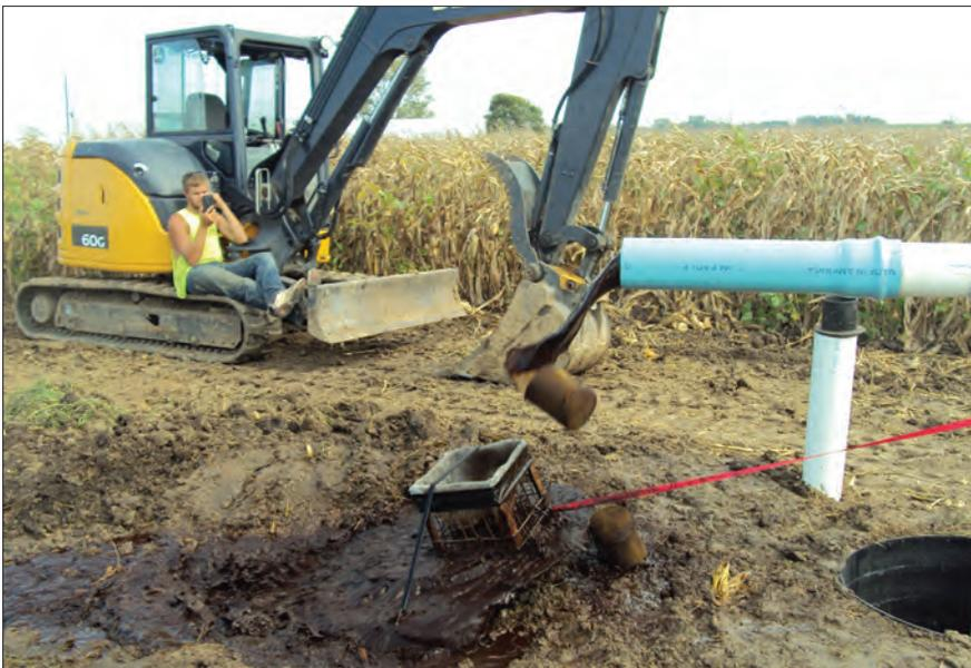
**And here they are! This photo shows foam swab "pigs" exiting the water main. The flow rate was 265 gpm in order to achieve a three-foot per second flow velocity.**
