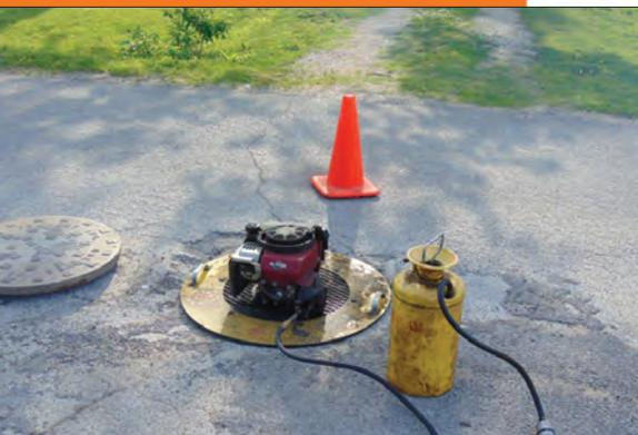
The smoke blower needs to set as flush as possible on the manhole to ensure no smoke escapes. Smoke is created by special oil dripping onto the engine muffler.
