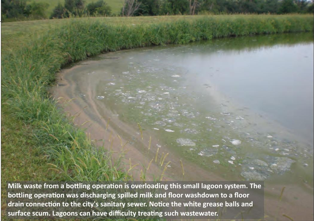
Milk waste from a bottling operation is overloading this small lagoon system. The bottling operation was discharging spilled milk and floor washdown to a floor drain connection to the city's sanitary sewer. Notice the white grease balls and surface scum. Lagoons can have difficulty treating such wastewater.
