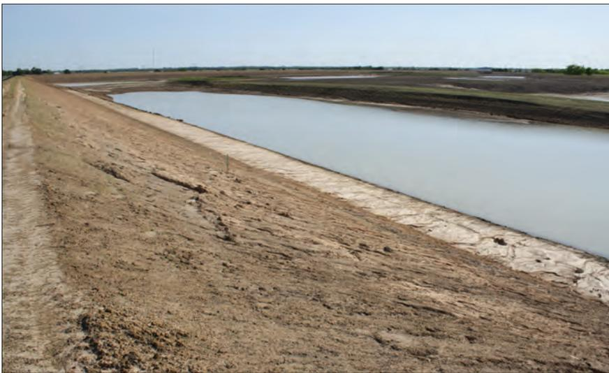
Portion of the Confined Disposal Facility where sediments will be redeposited and water will be allowed to clarify before returning to the Neosho River.
