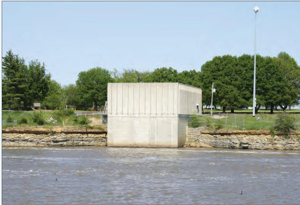
**Water intake facility for Wolf Creek Generating Station located downstream from John Redmond Reservoir on the Neosho River.**
