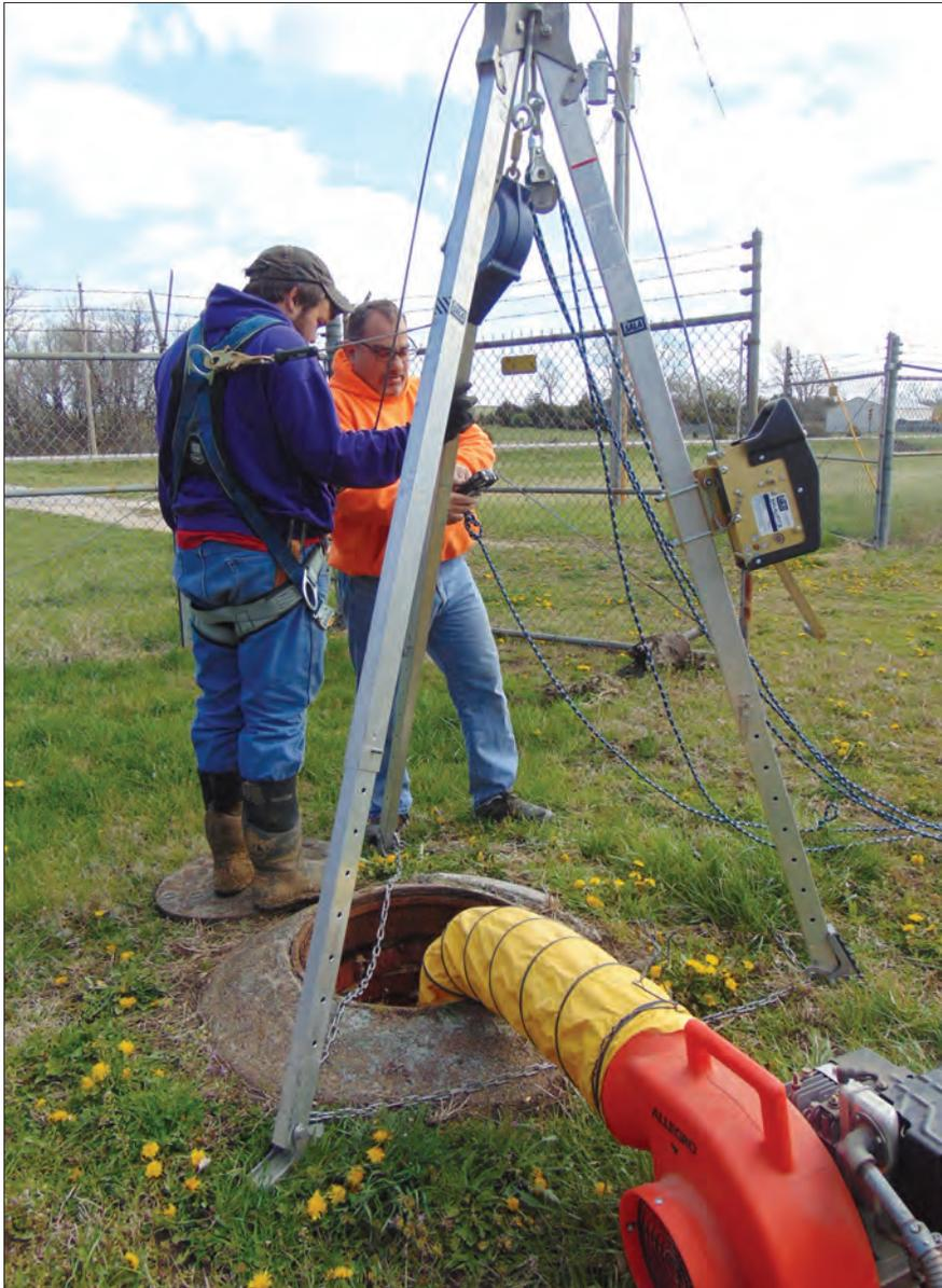
**Neil Clowe, Wetmore, Kan. is ready to enter the manhole to remove a sandbag left during construction of the lift station. Note fall protection connected to the back of the harness, raising line connected to the front of harness and 4 gas monitor in his left hand and ventilation fan all in place.**
