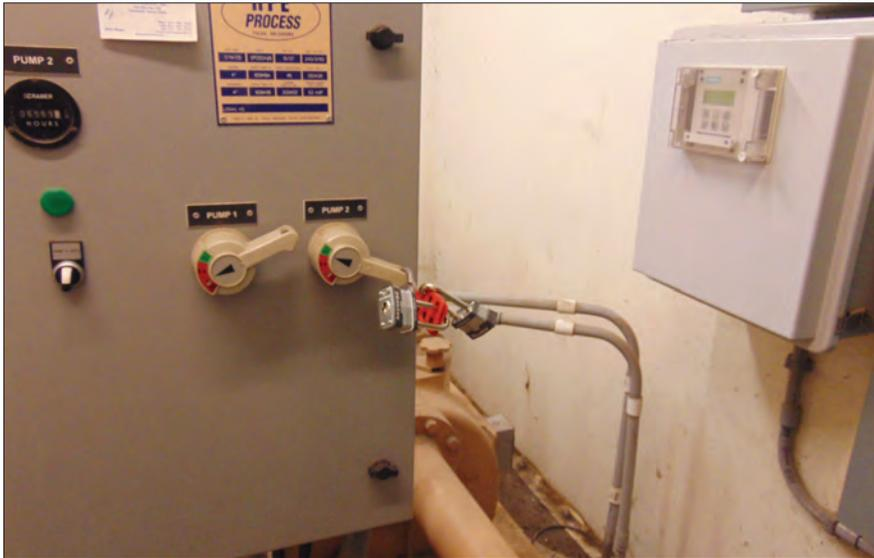
This photo shows the lockout/tagout installed by David Snow, city of Logan, Kan. to lock out the pumps at a lift station prior to adjusting the impeller clearances.
