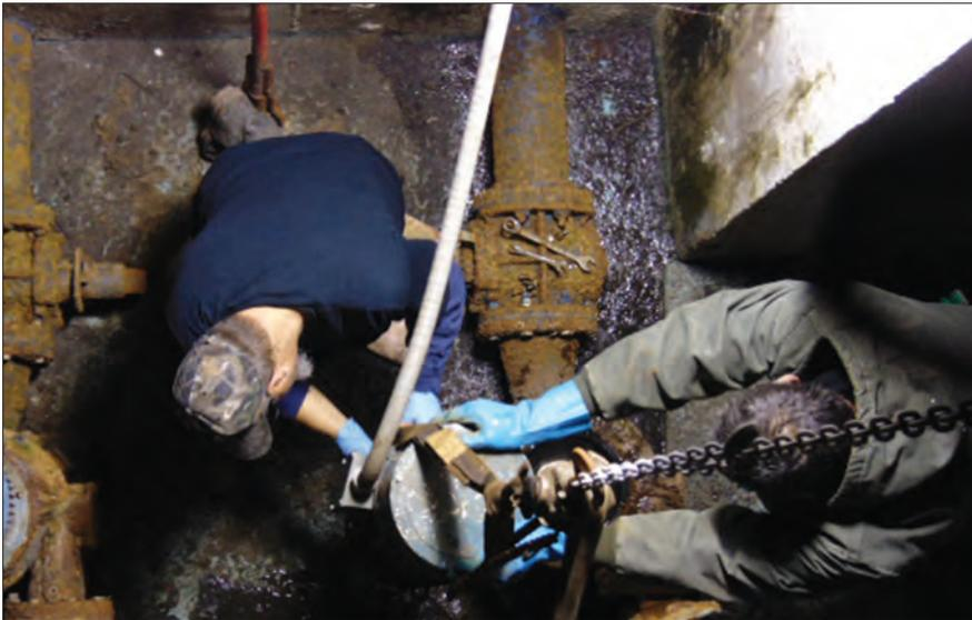
Staff at the City of Horton work to pull a pump at a lift station to remove a blockage. Note the heavy rubber gloves workers are wearing.
