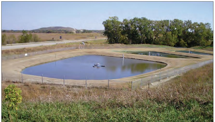
**This photo shows the same lagoon four months later after treatment with Diquat to control duckweed. This discharging lagoon was not meeting effluent limits while covered with duckweed. Once the duckweed blanket was controlled, the lagoon returned to compliance with all parameters.**
