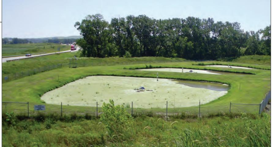
**Notice duckweed on all three lagoon cells and very little open water on the surface. Even solar mixers are not able to breakup the duckweed blanket.**
