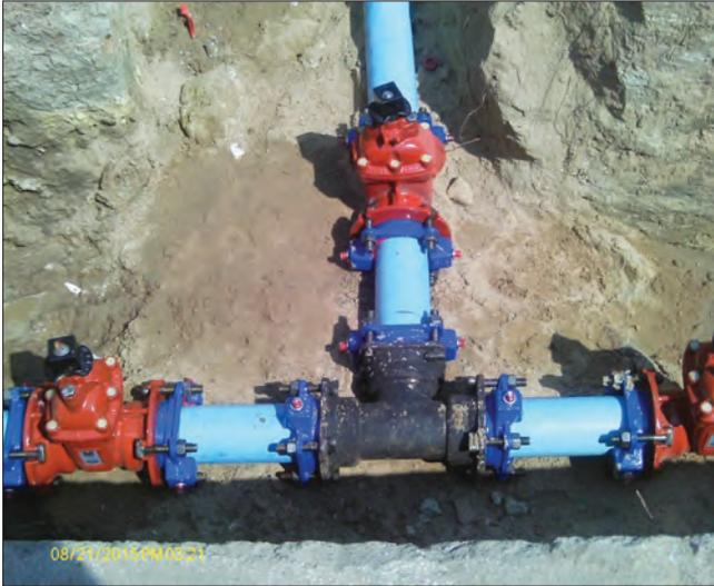
This close up of the drone picture shows that all fittings have restraint couplings.
