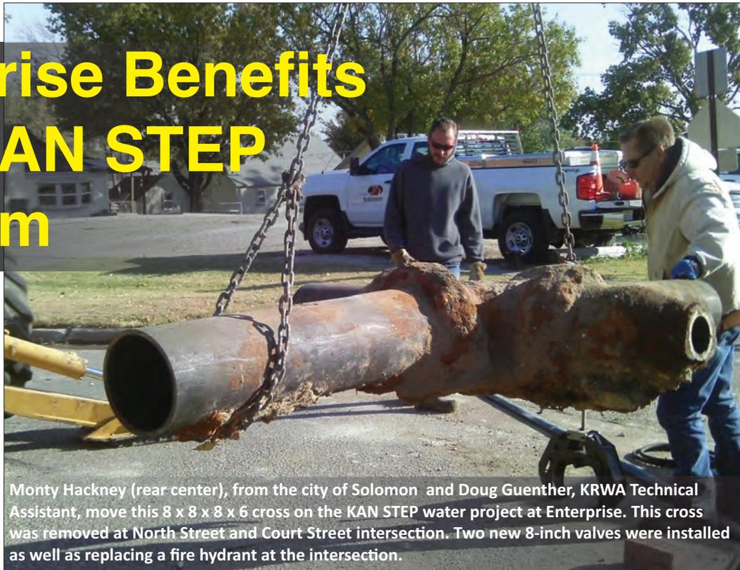
Monty Hackney (rear center), from the city of Solomon and Doug Guenther, KRWA Technical Assistant, move this 8 x 8 x 8 x 6 cross on the KAN STEP water project at Enterprise. This cross was removed at North Street and Court Street intersection. Two new 8-inch valves were installed as well as replacing a fire hydrant at the intersection.
