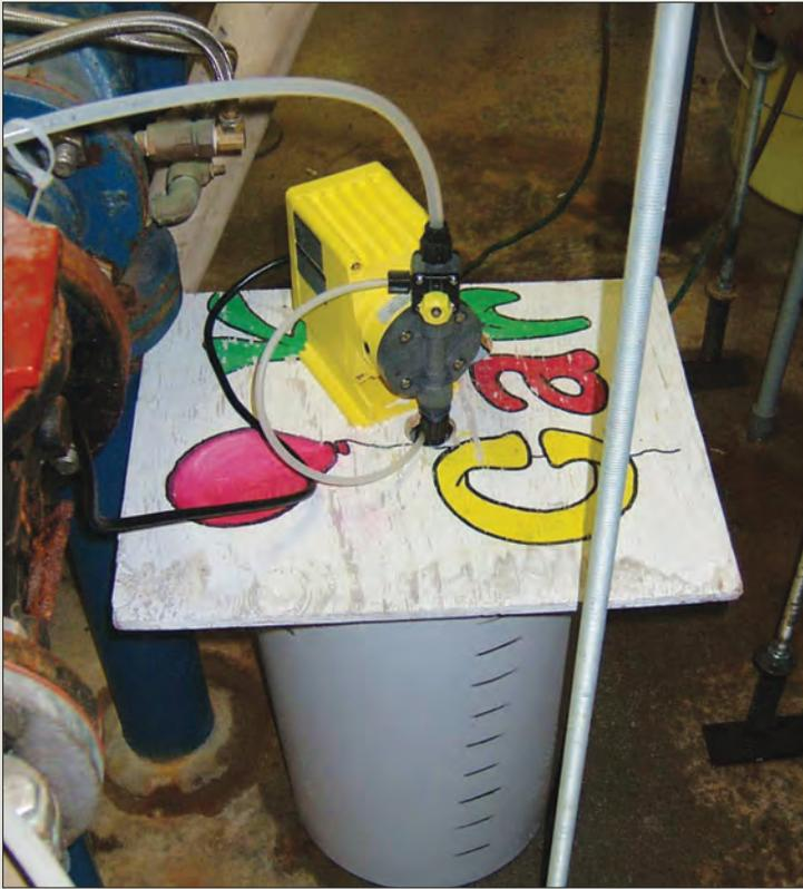
This ammonium sulfate feed system is for a very small 60 GPM flow at a rechlorination system at a pump house in a distribution system. Ammonium sulfate is purchased in 25 pound bags and mixed at only 0.25 pounds per gallon of feed solution. Rechlorination and ammonia addition are only needed in this system the summer and early fall months. The chemistry and the chemical reactions are the same regardless of the size of the feed systems.
