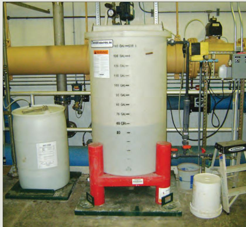
This photo shows ammonium sulfate solution feed equipment for a 500 GPM water treatment plant. The solution is made from purchased granular ammonium sulfate in 25 pound bags. The solution strength is determined by the plant operators.
