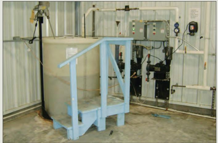
This ammonium sulfate solution feeding equipment is used in a 1,000 GPM water treatment plant. The plant purchases the solution already mixed.
