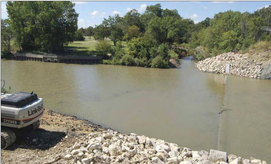
**From the east bank above the opening of the cut-off channel (from left to right), one can see the surface water intake in Bill Burke Park, the original Smoky Hill River channel where it turned to the west into the city of Salina, and the new scour key crossing the opening of the cut-off channel.**
