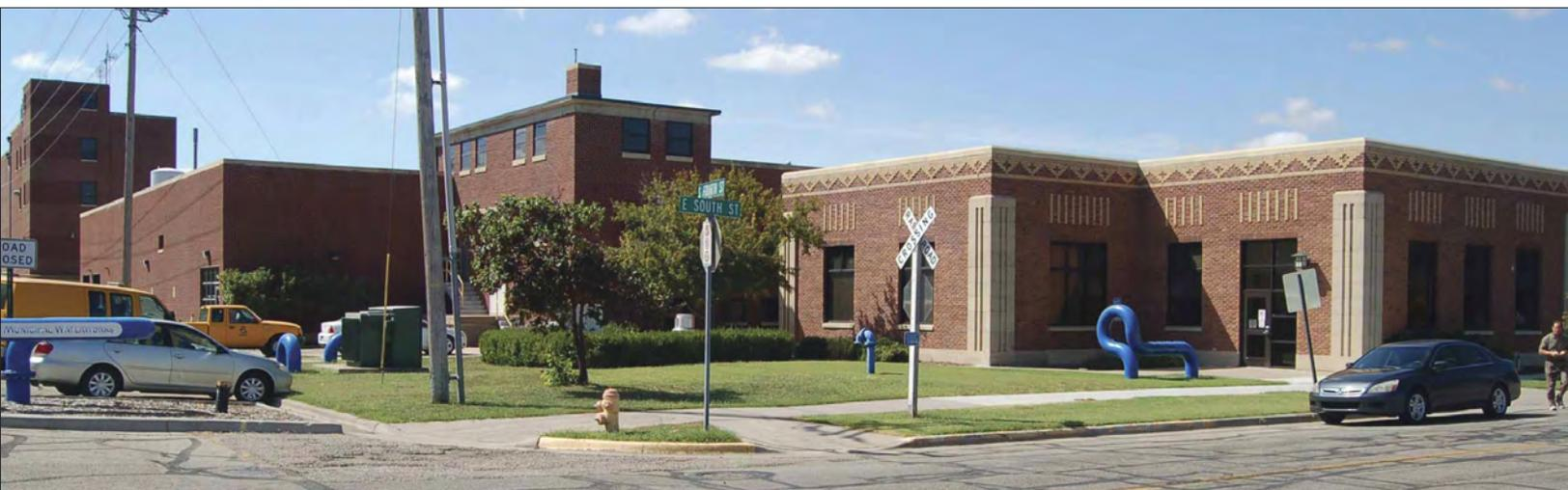
The Salina water treatment plant is located near the downtown district, on the bank of the old Smoky Hill River channel. The plant has air-stripping, settling, softening, filtration and disinfection processes that produce high quality drinking water from surface water and groundwater.
