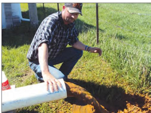
**Cleaning the 2.5 miles of 6-inch PVC pipeline removed a lot of sediment from the interior of the line. Most of the sediment was a very fine sand and the color of the discharge indicates that iron and manganese are also in the water.**
