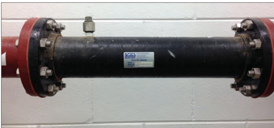
This is the Koflo static mixer installed to provide improved mixing. A stainless steel element inside the pipe spool will cause rapid mixing of the two well waters to lower the selenium concentration in the finished water.
