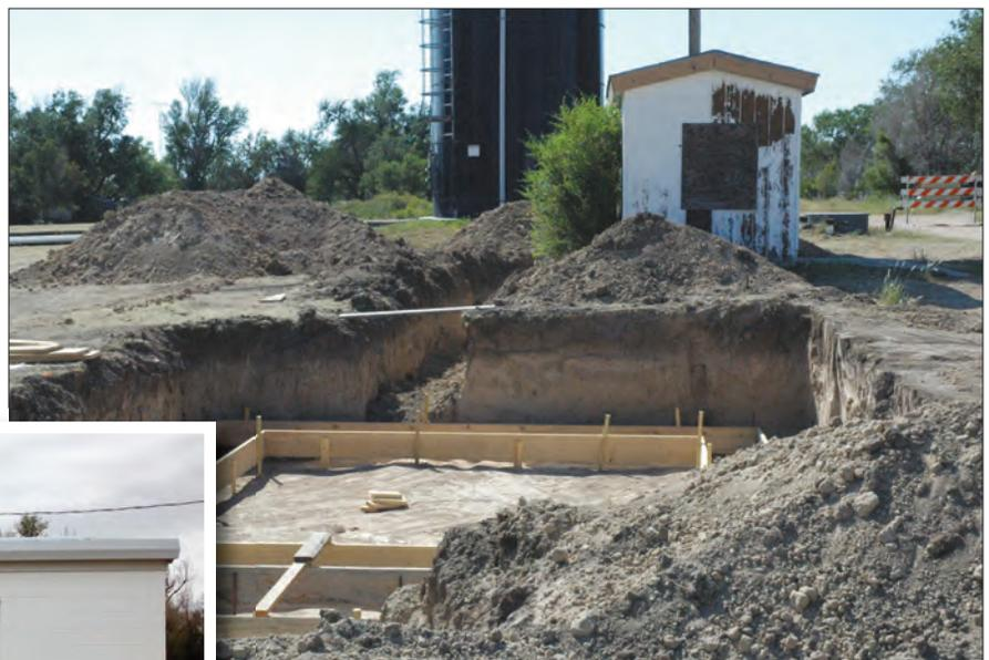
These photos show various stages of the construction of the new blend/chlorination building. Note the standpipe and old booster pump building in the background. The old building will be removed.
