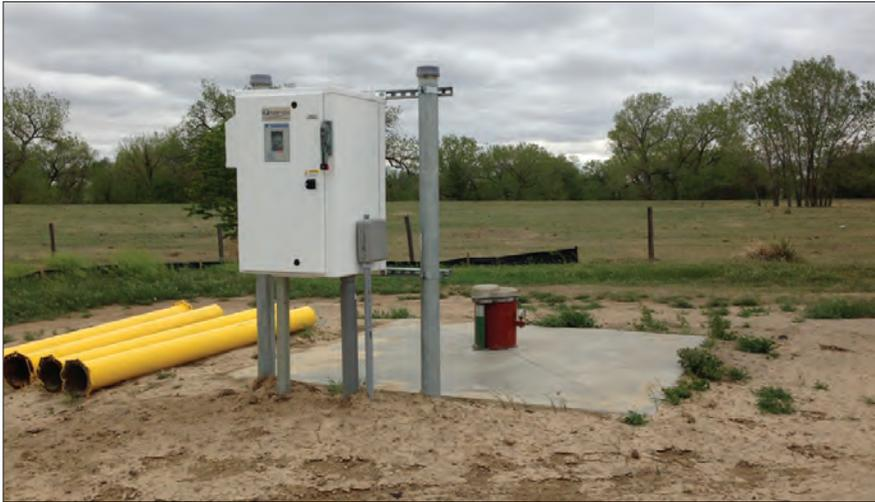
This photo shows the new well at the southeast edge of town. This well and the existing well in this area will be used to blend down the selenium from the north well. The four yellow metal posts laying on the ground will be installed around the perimeter of the well for protection.
