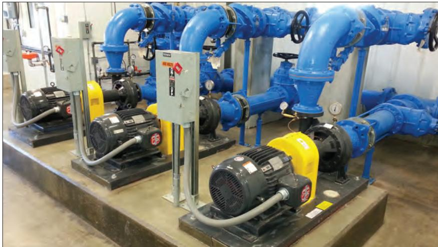
Three, 600 GPM high service pumps in the new water treatment plant at St. John, KS are controlled by variable frequency drives.
