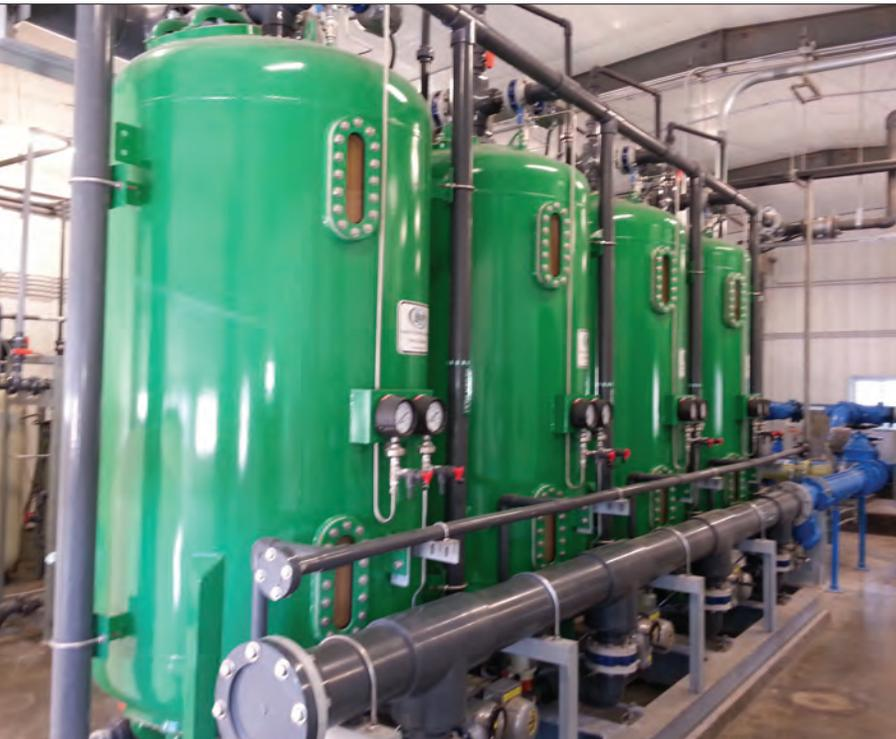
The photo at left shows the four, skid-mounted treatment vessels to remove nitrate from groundwater. Incoming nitrate is 12 mg/L. Water is treated and then blended to provide a finished water in the 7 to 9 mg/L range.
