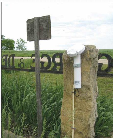
IDT Harmony® satellite reading antennae mounted on backside of rock post.
