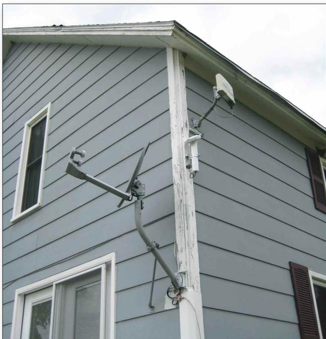
**The corner of this house in Washington RWD 1 has three antennae, with the center unit being the IDT Harmony® water meter reading technology.**
