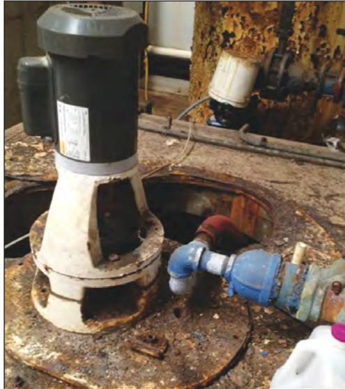
Treatment plant piping and appurtenances need to be wire-brushed, corrosion removed and painted.
