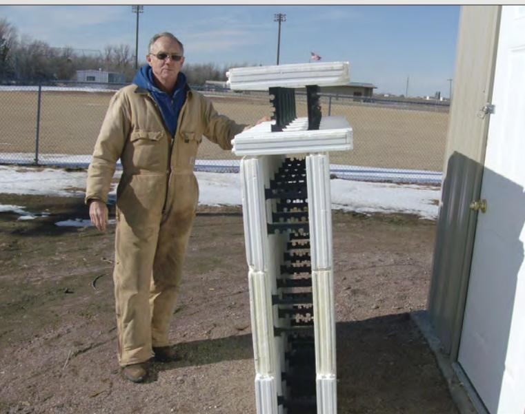
Jerry explains the concrete form system used on the sidewalls of new well building.
