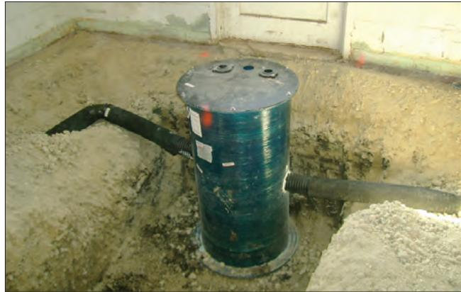
**This sump pit and tile were installed around the perimeter of the Udall Community Center to alleviate water build up under the new concrete floor. A slab will also be poured between the community building and the neighboring building to the north to divert rainwater towards the street west of both properties and away from the buildings.**
