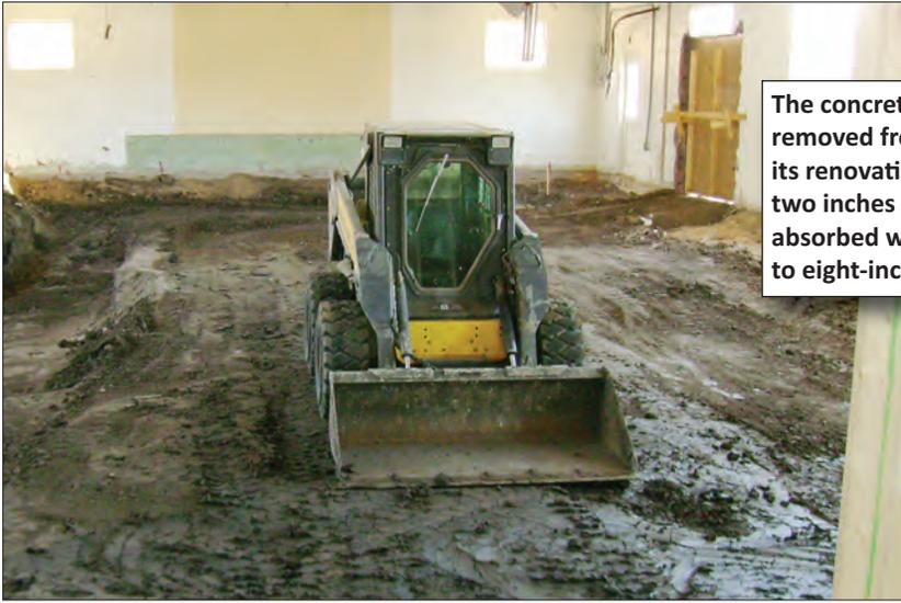
The concrete floor and nearly four feet of soil was removed from the Udall Community Center as part of its renovation. The original floor had heaved nearly two inches as “fatty clay” soil under the floor absorbed water. AB3 was hauled in and packed in six- to eight-inch lifts.
