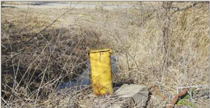
**This monitoring well, in the area of the industrial wells, appears to have been damaged by agricultural or construction activities, and may be unusable for water level measurements or water quality testing. This lack of maintenance, combined with no water use over five years, would likely be strong evidence in an abandonment hearing.**
