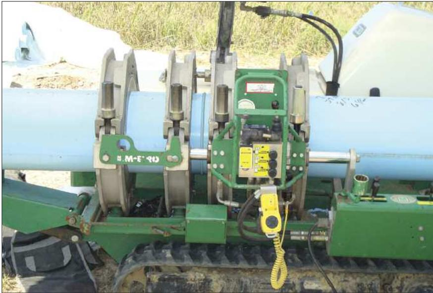
The contractor on the project, J and K Contracting, Junction City, KS, fused the new pipe using this McElroy Tractstar fusion machine.
