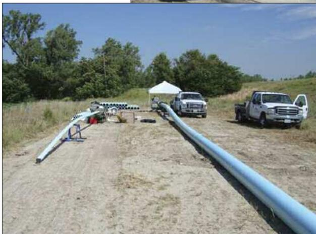
**Concordia opted to install a 10-inch fusible PVC pipeline for the extension north of the city. The pipeline crosses the Republican River. A unique feature was the addition of a 4-inch PVC line was also installed as a return to recirculate the water in the system.**
