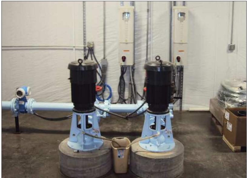
These new high service pumps were equipped with variable frequency drives to help control the plant and also eliminate water surges on the system.
