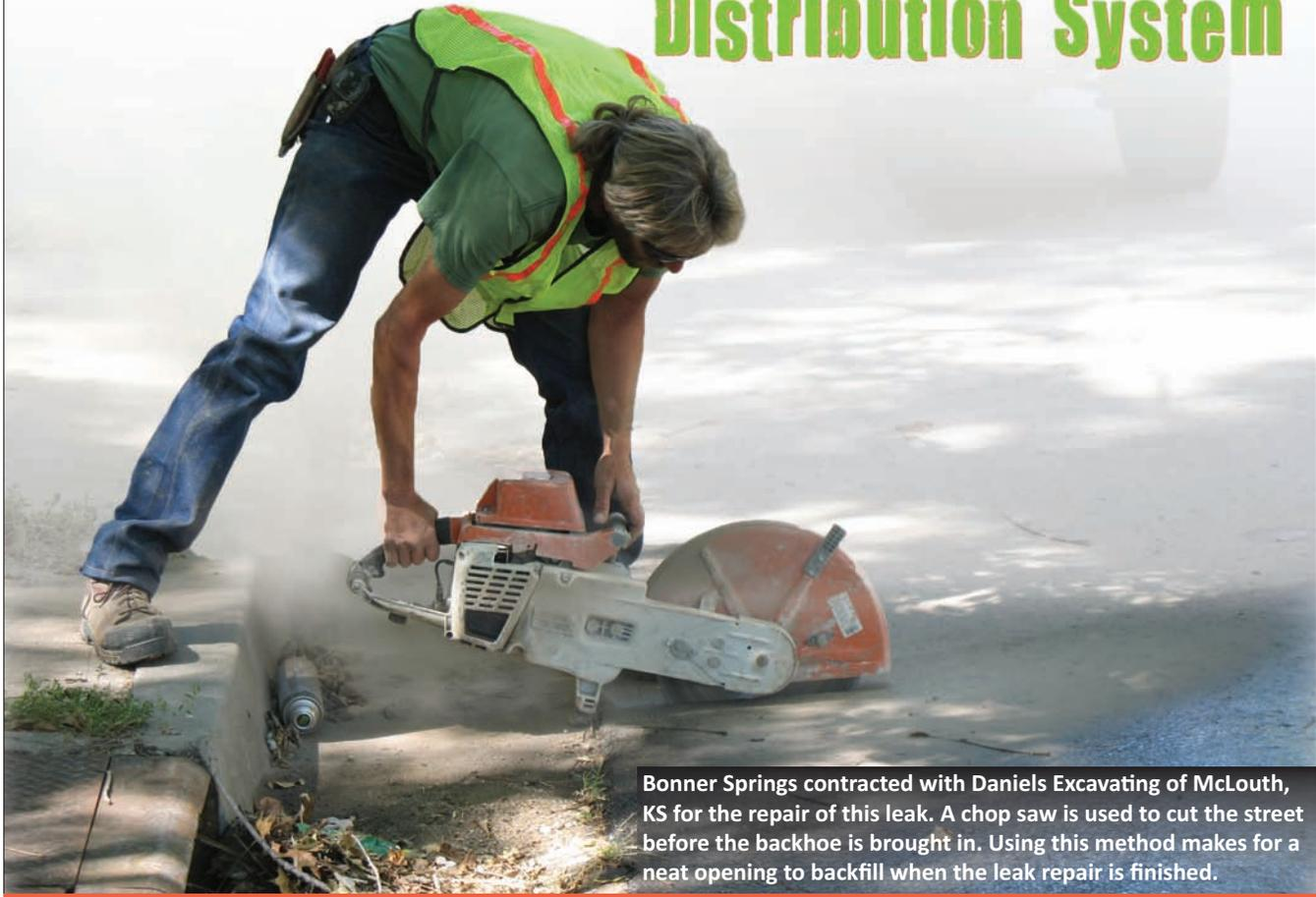
Bonner Springs contracted with Daniels Excavating of McLouth, KS for the repair of this leak. A chop saw is used to cut the street before the backhoe is brought in. Using this method makes for a neat opening to backfill when the leak repair is finished.
