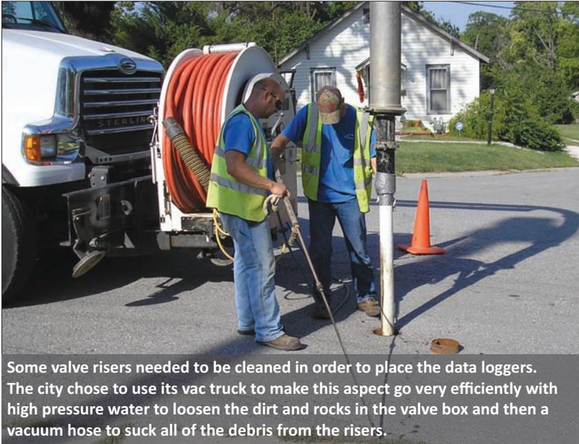
Some valve risers needed to be cleaned in order to place the data loggers. The city chose to use its vac truck to make this aspect go very efficiently with high pressure water to loosen the dirt and rocks in the valve box and then a vacuum hose to suck all of the debris from the risers.
