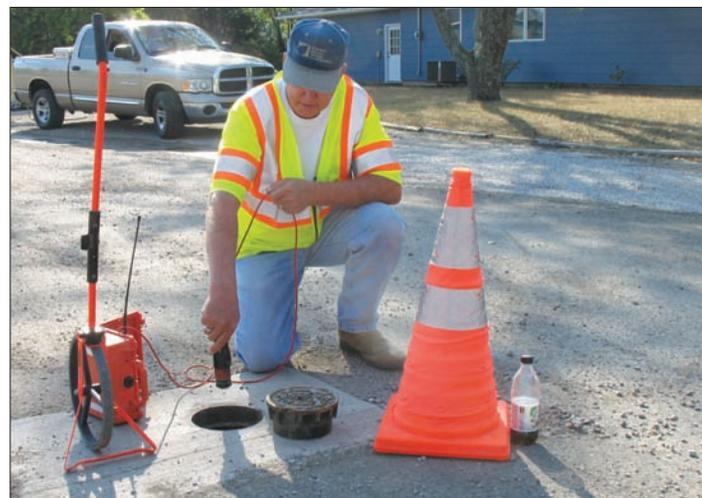
**KRWA Tech Gary Armentrout lowers one of the two microphones used to correlate the location of a pipeline leak onto a valve. If all of the information entered into the computer is correct, the correlator will locate a leak to within six inches.**
