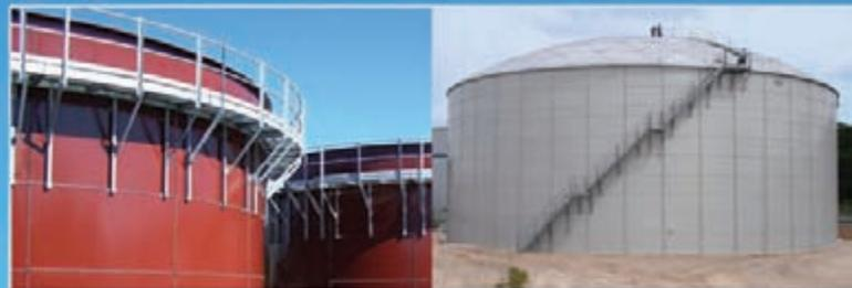
Tank Connection is the only tank supplier that designs, manufactures and installs all four types of steel storage tanks including RTP, field-weld, shop-weld and hybrid tank designs for potable water storage. Our precision RTP (rolled, tapered panel) construction is the #1 bolted tank design selected worldwide.
