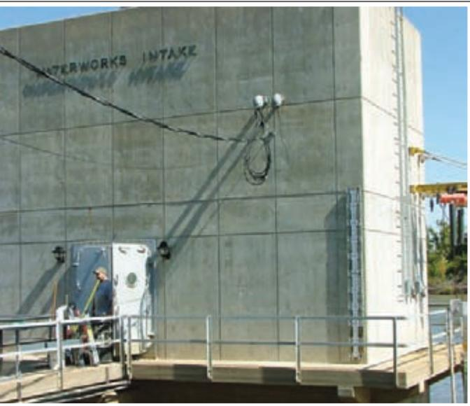
The Navy ship door that was installed years ago prevented flood water from entering the north plant intake structure. Also note the ladder on the side of the structure that was used by city staff to gain entry during the flood.
