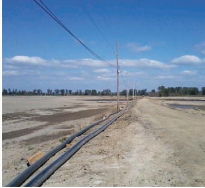
These pipes are a part of the emergency pumping system used to move surface water to the South Plant.
