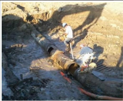
This photo shows a cut being made in the 24-inch transmission line north of the channel scour taking out 340 feet of 24-inch line. The purpose of the cut was to install a by-pass around the failed section of transmission line using 2 parallel lines of 8-inch HDPE pipe. The by-pass is now operational and is allowing us to pull water directly from our wells and deliver the water to the South Plant for treatment.
