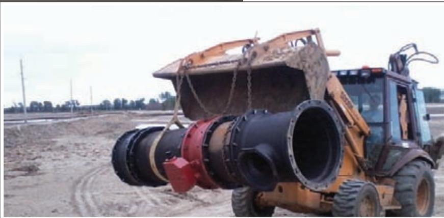
A worker moved a pipe section with isolation valve into place to prepare for possible flood damage. This valve was eventually closed to prevent surface water from flowing back to the wells when the emergency system which was pumping surface water was activated.
