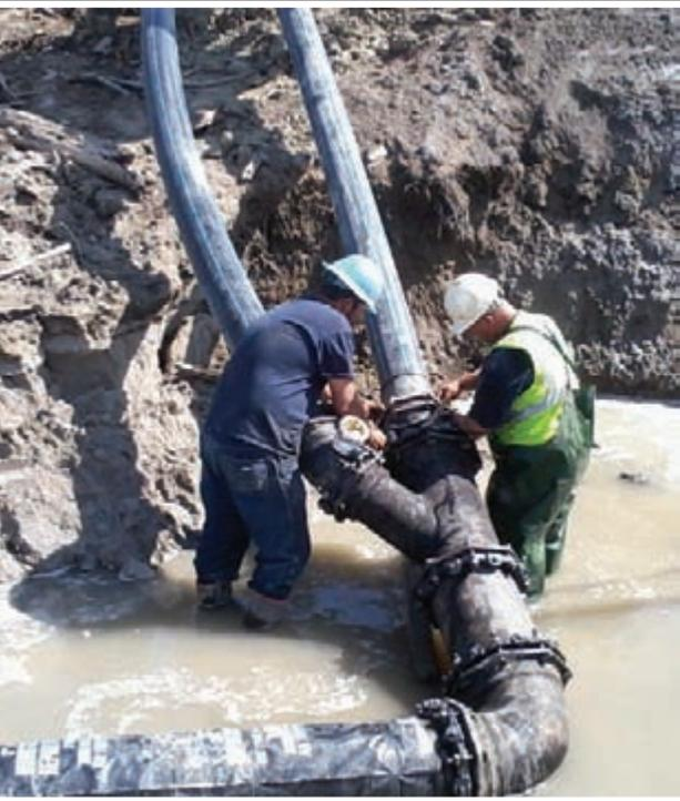
This photo shows the connections for the by-pass system that is now operational and allowing us to pump ground water from the wells to the South Plant. The surface water diversion and pumping system served its purpose is being dismantled.
