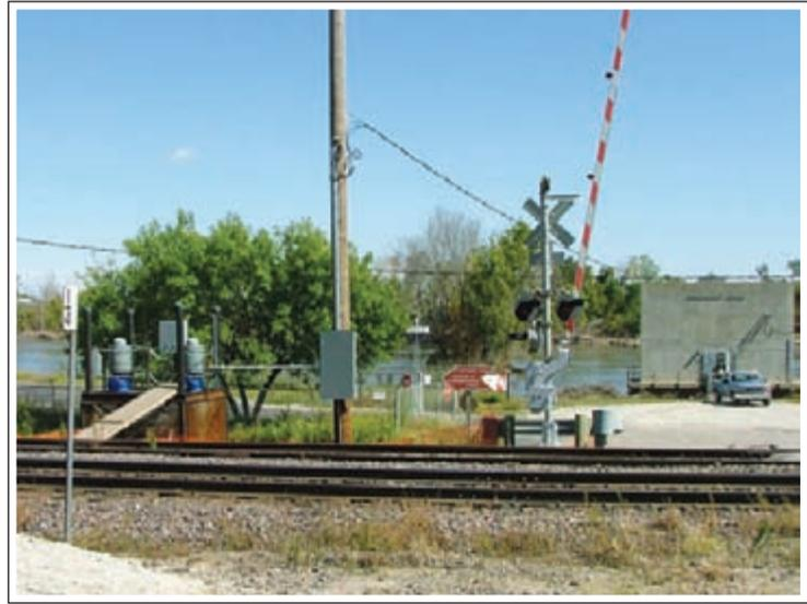
This photo shows the relative location of the intake structure to the emergency pumping station for the North Plant. The emergency pumping station is in the foreground near the Union Pacific RR Tracks. The emergency pumping station performed adequately when test operated but was not needed because even though all three raw water pumps were under water, one continued to operate delivering water to the plant.
