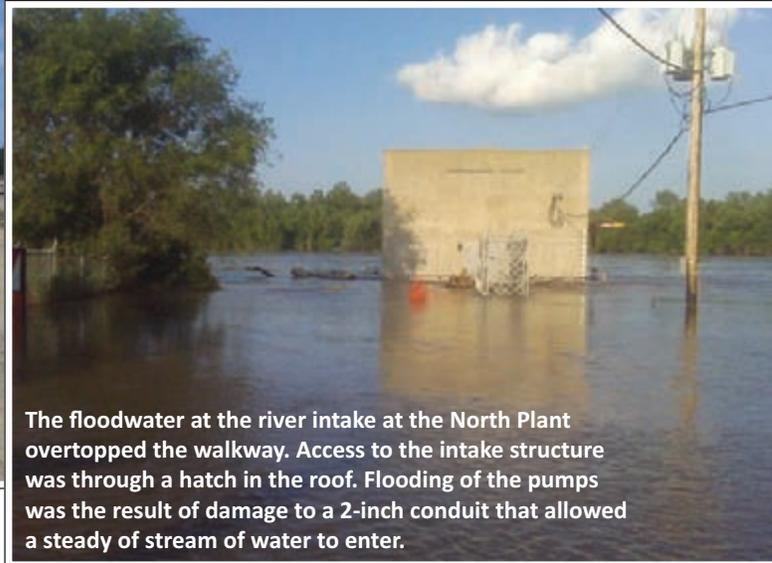
The floodwater at the river intake at the North Plant overtopped the walkway. Access to the intake structure was through a hatch in the roof. Flooding of the pumps was the result of damage to a 2-inch conduit that allowed a steady stream of water to enter.
