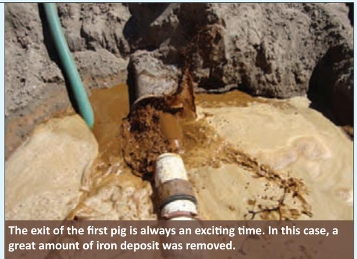
The exit of the first pig is always an exciting time. In this case, a great amount of iron deposit was removed.
