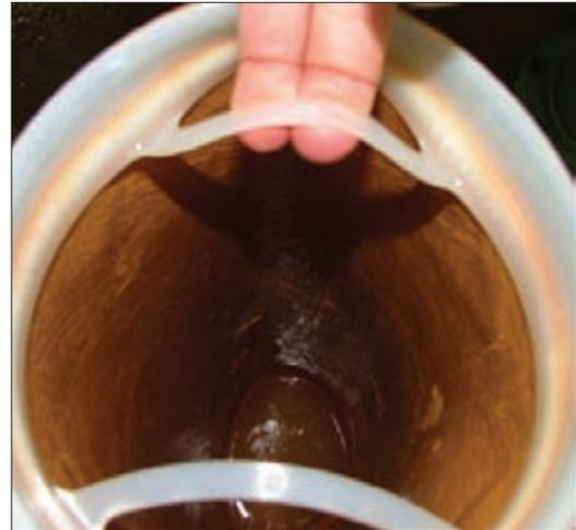
This photo shows the center of the bag filter with iron accumulation.
