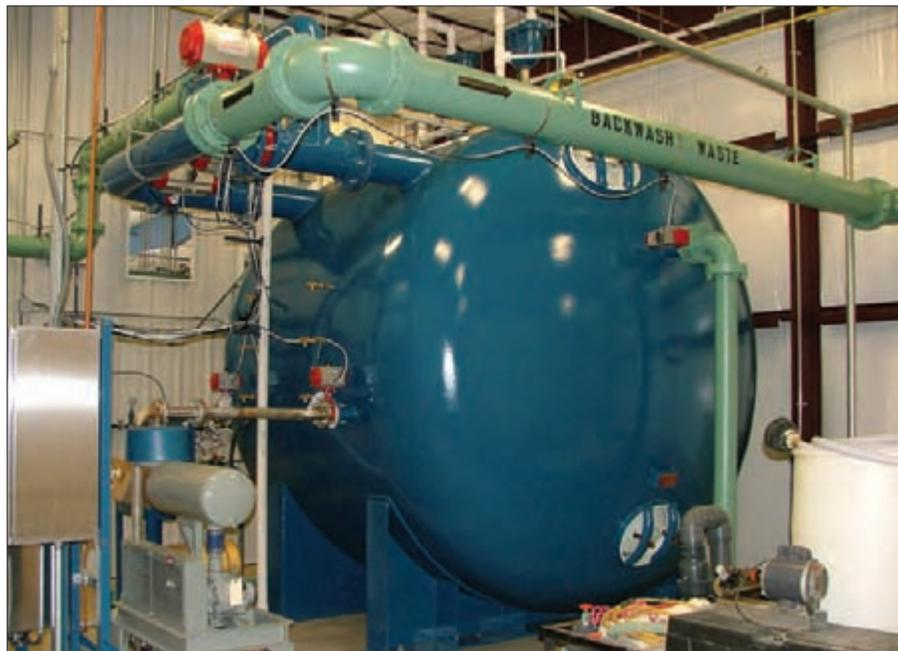
This is the two-cell pressure sand filter that was installed to remove oxidized iron and clay particles before reaching the Hydrex cartridges and RO membranes. This unit is the main focus of this improvement project.
