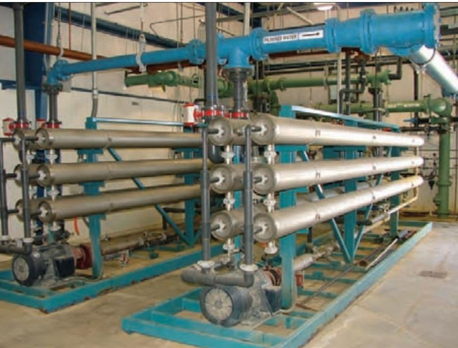
This is an end view of the two RO skids. The RO membranes were recently replaced after about 9 years of use at a cost of \$72,000.
