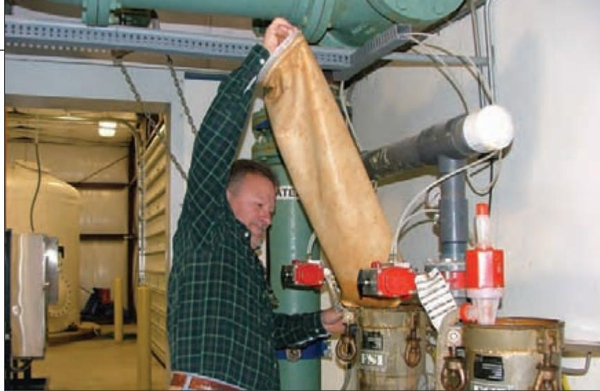
Dan Hoobler, operator, is removing a bag from the canister. Note the brown stain on the filter indicating iron was removed from the raw water bypass (blend) line. Without the bag filter, the iron would have been allowed to enter the storage tanks and possibly the distribution system causing customer complaints. The bag filters will no longer be needed with the use of the pressure filter.
