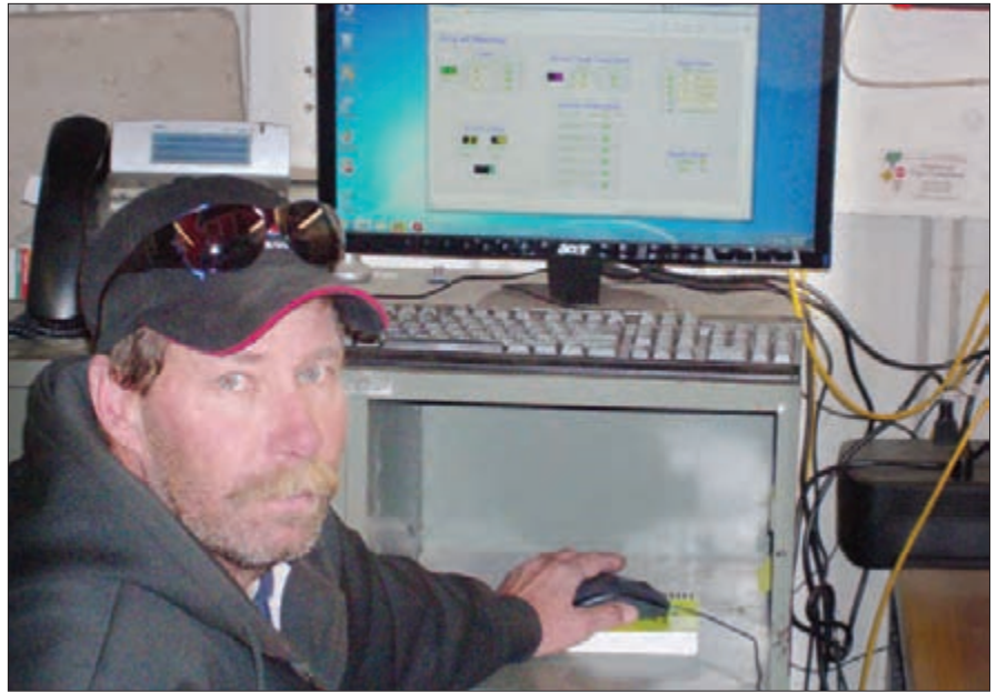
Manager Dan Bliss demonstrates the operation of the new radio telemetry and SCADA system.
