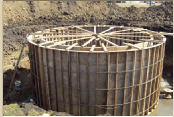
Caldwell Tank, Inc., Louisville, KY constructed the 50,000-gallon water tank. This photo shows the work on the foundation.
