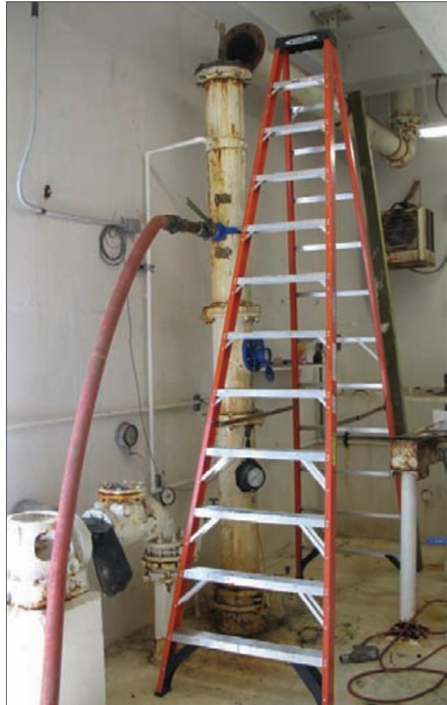
Where there is a will there is a way to test a large meter. A 90-degree elbow was removed from the top of this pipe and a plate was installed, then a 2-inch tap was made so this meter could be tested.
