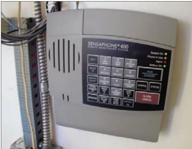
The city's Sensaphone 400 Remote Monitoring System monitors the water system for high or low chlorine residuals, chlorination system failure and power outages. If a warning is detected this system immediately notifies city staff so they can respond promptly.
