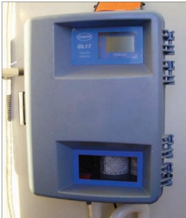
The city's Hach CL-17 Analyzer monitors free chlorine residuals continuously at the POE. The analyzer is also equipped with a dialer system. While Enterprise's population is not large enough to require continuous residual monitoring, the city wanted to make sure operating staff would be notified if residuals were too high or too low.
