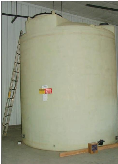
This tank store sodium chloride (salt). Salt is used to re-generate the anion exchange resin in the five exchange tanks.
