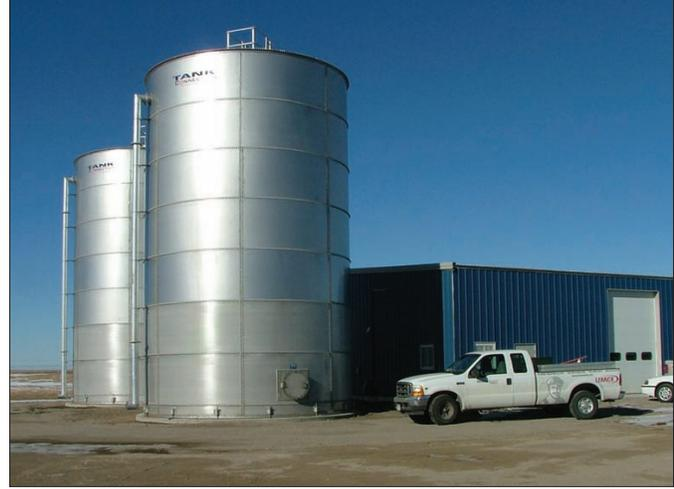
This metal building houses the treatment plant; the two stainless steel tanks are used to store treated water. Each tank has a capacity of 100,000 gallons.
