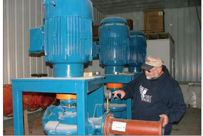
Rich Simon, Water Superintendent, points out the need and use of the pressure gauge at one of the three high service pumps. These pumps pick up treated water from the stainless steel tanks and deliver it to the distribution system. Note the piping is not yet connected in this photo taken in early January 2011. This project is not yet completed. The target completion date is March 1 and April 10 is the deadline for the plant to be operational.
