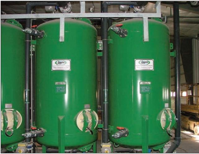
This photo shows two of the five ion exchange units supplied by Layne Christensen Company. The tanks contain nitrate selective resin for nitrate removal and are the main workhorse in the water treatment plant.
