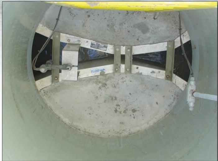
Wastewater weir with flow sensing equipment installed
