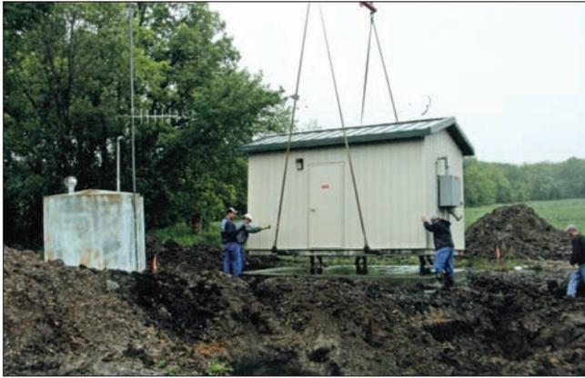
A crane crew sets the new booster pump station; the station replaces an original station installed in 1974.
