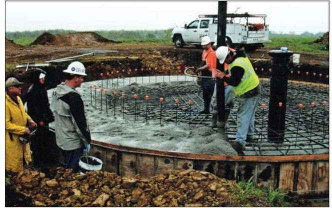
A crew for Engineering American pours concrete for the base of the new 200,000-gallon water storage tank.
